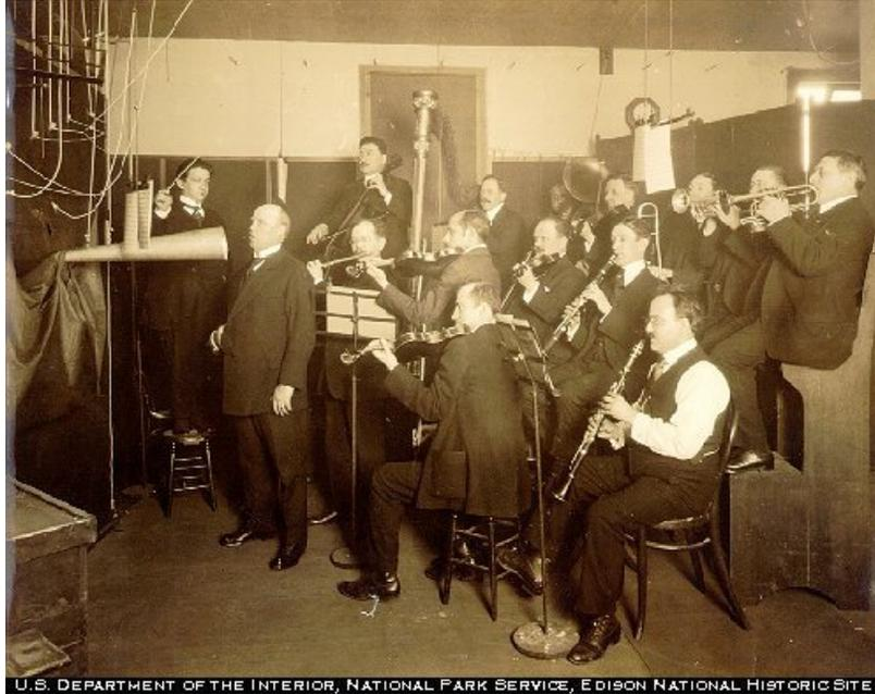
Figure A2-5: Recording at the Edison Studio, 79 Fifth Avenue, New York City, Jacques Urlès singing, Sodero conducting, March 30, 1916. Note the narrow conical horn of approximate length 1 m in use. Photo courtesy of the Edison National Historic Site, used by permission.
